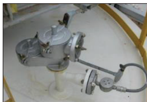
Pressure Vacuum Relief Valve
